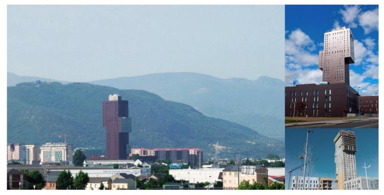
"La Rosaleda" Tower, is an outstanding high rise building (100 m) set within a larger project which includes a hotel, car parks, offices and residential housing. The total surface area to be constructed is 40,140 m<sup>2</sup>, 40 % of which belong to the 30 floors of 20 x 24m of the standard section of the tower.
